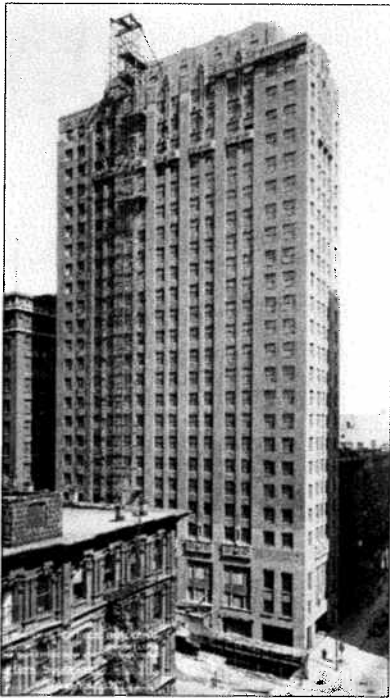
A construction photo of the Old Dearborn Bank Building, c. 1928. The Building is an unusual mixture of exotic terra cotta and warm-hued bricks used on a tall, narrow Art Deco skyscraper.
